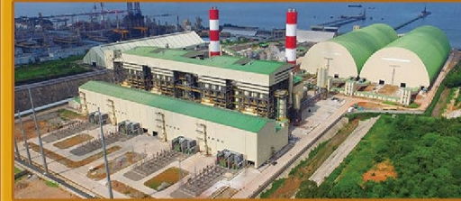
Therma South Inc. TSE-1 Davao, Philippines CFB 520 T/H X 150 MW X 2
