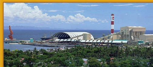
Toledo Power Company TPC-1A Cebu, Philippines CFB 300 T/H X 82 MW
