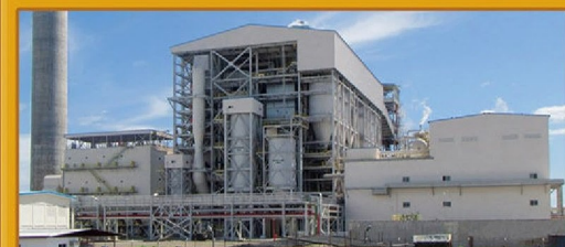
Therma South Inc. TSE-1 Davao, Philippines CFB 520 T/H X 150 MW X 2
