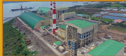
Cebu Energy Development Corp. CEDC Cebu, Philippines CFB 300 T/H X 82 MW X 3
