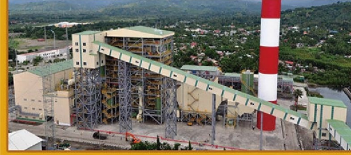
Taganito HPAL Nickel Corp. THP-1 Taganito, Philippines CFB 300 T/H X 48 MW
