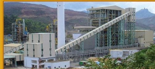
Taganito HPAL Nickel Corp. THP-1 Taganito, Philippines CFB 300 T/H X 48 MW
